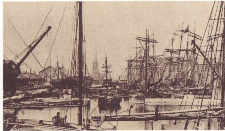
Busy Aldam Dock in the late 19th century
