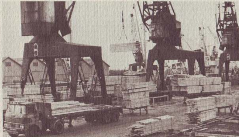
74 tonne quay cranes discharging Swedish timber to importers' vehicles and stillages
